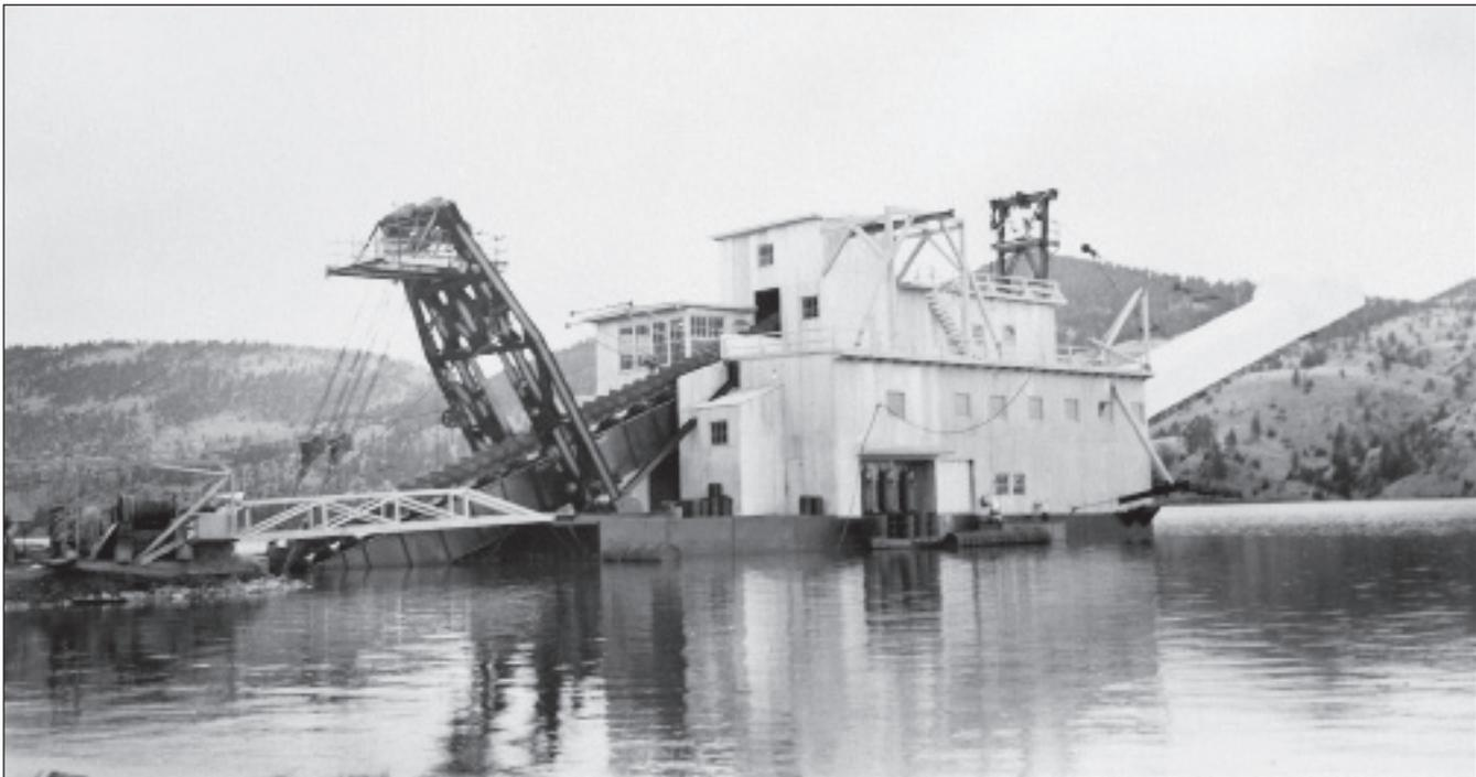
Figure 3. The Perry Schroeder Mining Company's dredge mining sapphires and gold on Eldorado Bar. The buckets are on the digging ladder to the left and the stacker is in the white covering on the right. Photo from the Photograph Archives, Montana Historical Society, Helena, MT.
