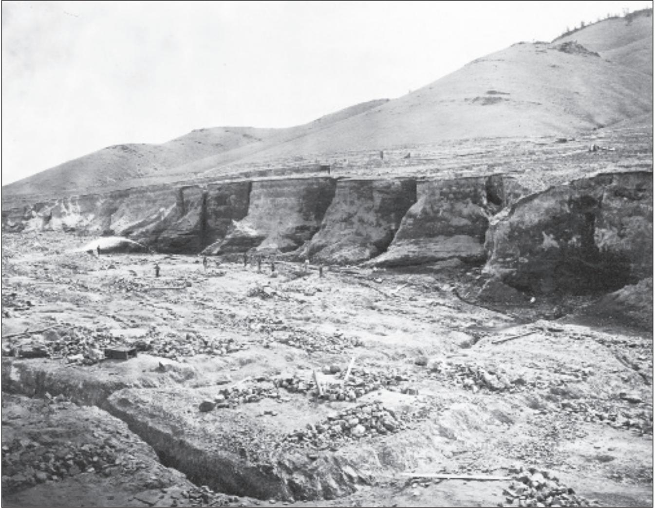
Figure 4. Photo of hydraulic mining at French Bar showing a monitor to the left and, barely visible, the hose bringing water down from the ditch above. Alluvium that forms the cliffs was stripped from the area in the foreground by ground sluicing. Photo from Photograph Archives, Montana Historical Society, Helena, MT.
