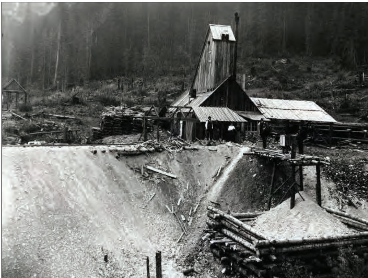
Figure 2. Tarbox mine, shaft headframe. Photo taken approximately 1900. From archive of Mineral County Historical Society, Superior, Montana.
