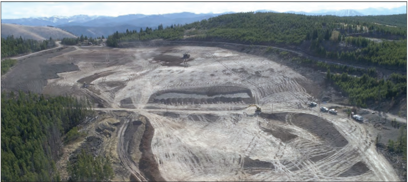
Figure 6. Photograph from the Montana DEQ showing the construction of the waste repository where the mill tailings and waste rock were buried.
