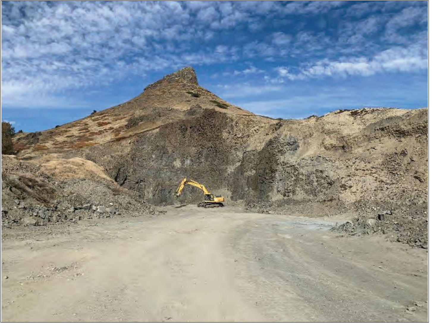
Figure 6. Shonkinite quarry near Fort Shaw, Shumaker Trucking and Excavating Contractors, Inc.
