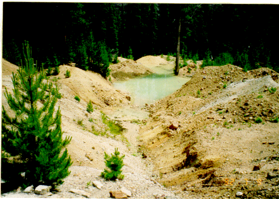
Figure 4A. After spring runoff and precipitation events, water ponds in the lower end of the cat cut.
