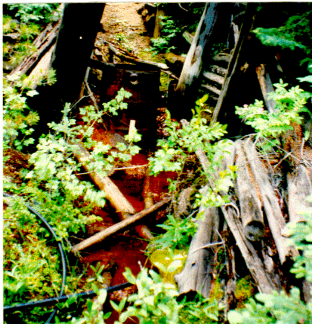
Figure 25A. The collapsed adit of the Phantom mine discharged water to Cataract Creek. Ferric hydroxide precipitate was evident for most of its length.
