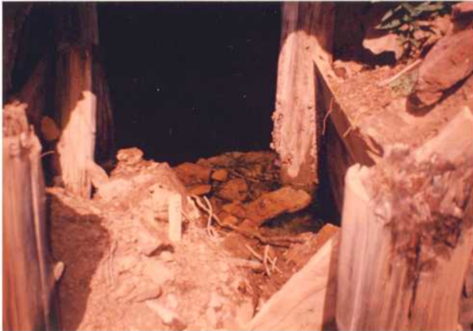
Figure 3.5 A small, clean discharge flows from open adit A-1. The discharge infiltrates the ground before reaching the creek.
