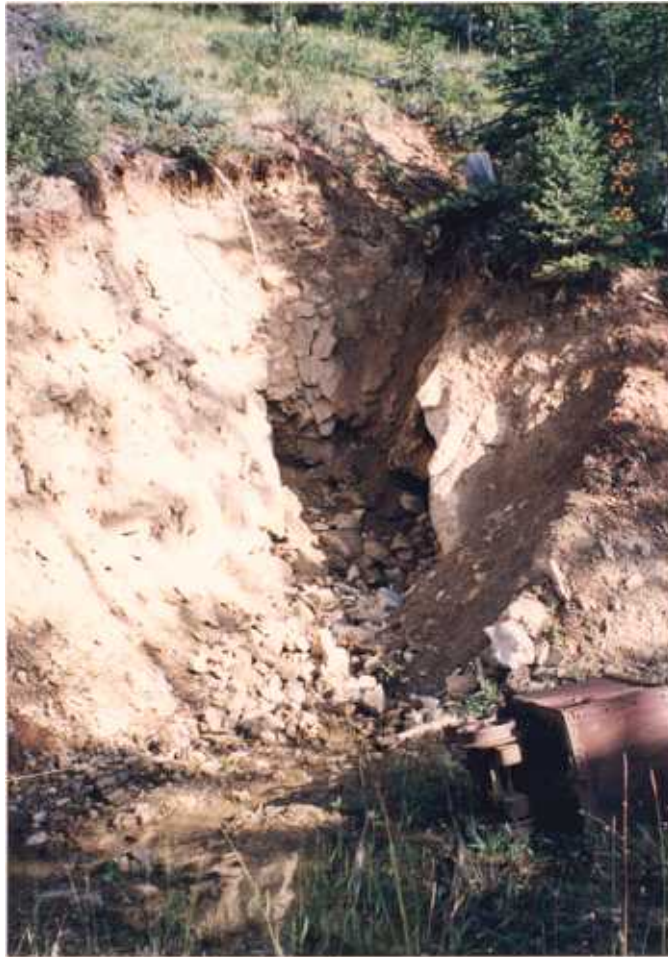
Figure 2.6 The Garrett mine has a single adit that discharges less than one gpm. Impact to the area appears to be restricted to the adit and waste-rock dump.
