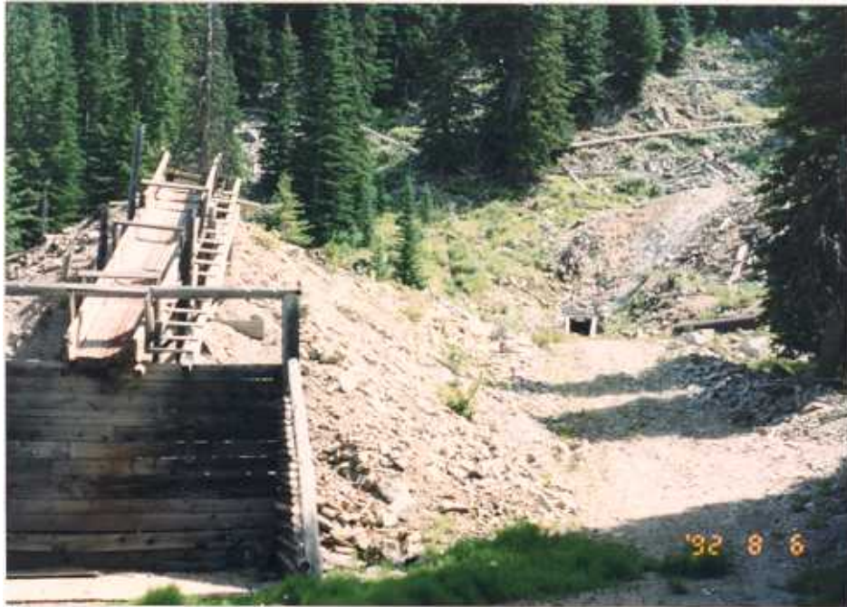
Figure 2.23 A spring breaks from the hillside above the adit of the Blue Bird mine. The adit also discharges water.
