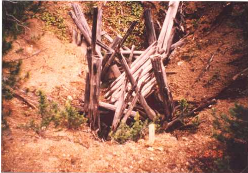
Figure 3.21 Flooded shaft S-3 is surrounded by a small waste-rock dump.
