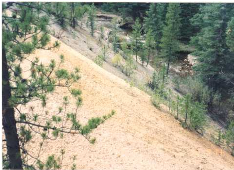
Figure 3.11 The Middle Fork of Rock Creek (upper right corner) is undercutting and eroding the sparsely vegetated waste-rock dump.
