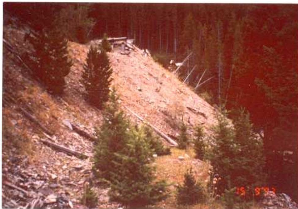
Figure 2.29 Grasses and conifers have taken root on the steep slopes of the waste-rock dump.
