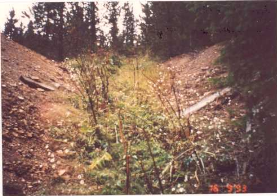
Figure 2.2a The discharge from the lower adit runs down the face of the waste-rock dump and into Harvey Creek.
