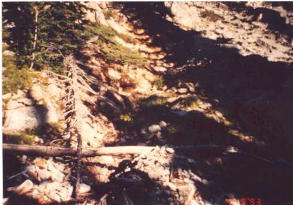
Figure 2.12b The A1 adit at the Ophir Mine is collapsed.
