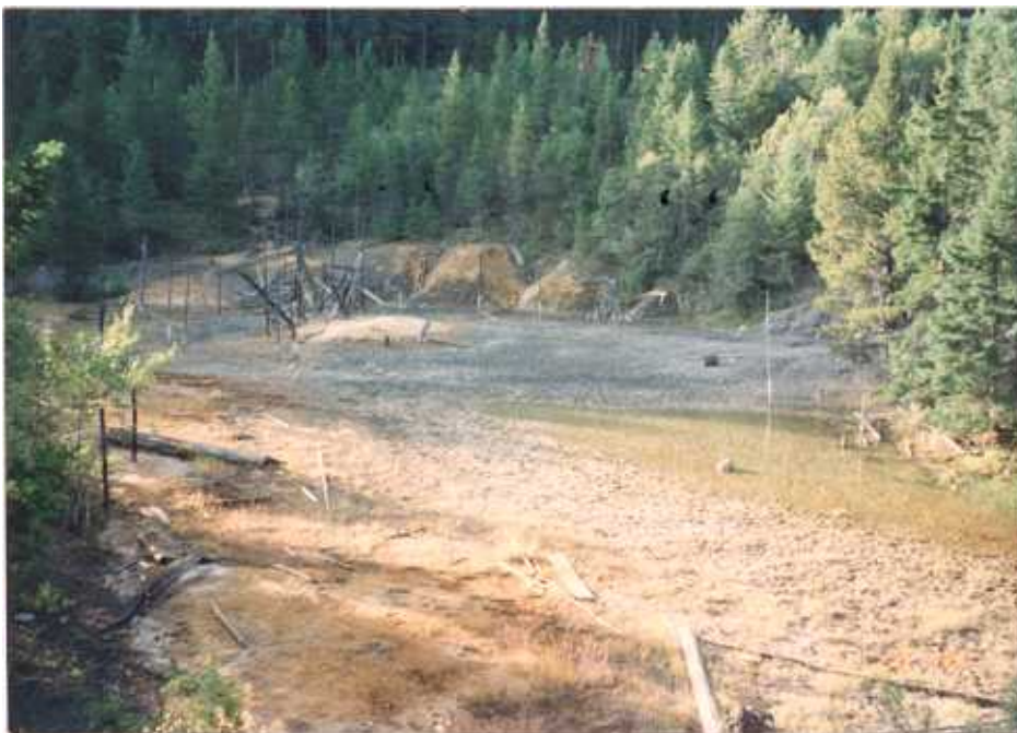
Figure 2.6b Lower tailings impoundment. A small seep west of the site feeds the pond. View is to the south west.
