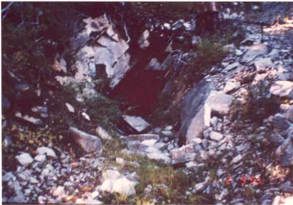
Figure 2.9b The A1 adit at the Independence Mine intact but flooded.
