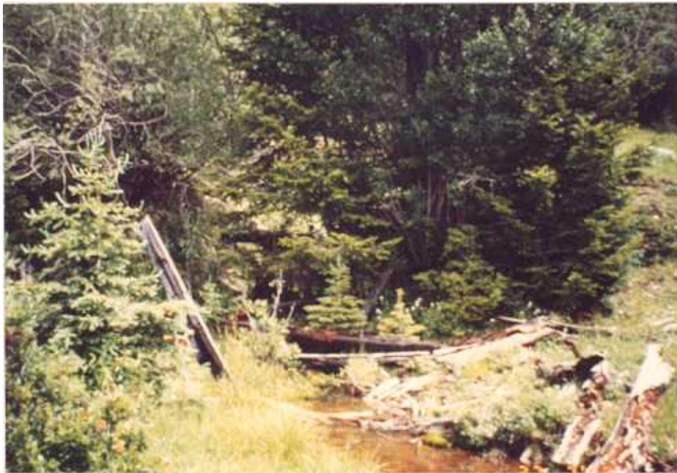
Figure 2.8b A substantial discharge flows from the collapsed main adit. The discharge is the headwaters of Basin Creek.
