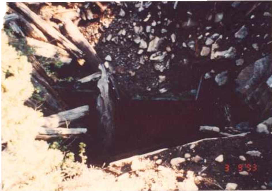
Figure 2.4a The S1 shaft flooded to within approximately five feet of the ground surface
