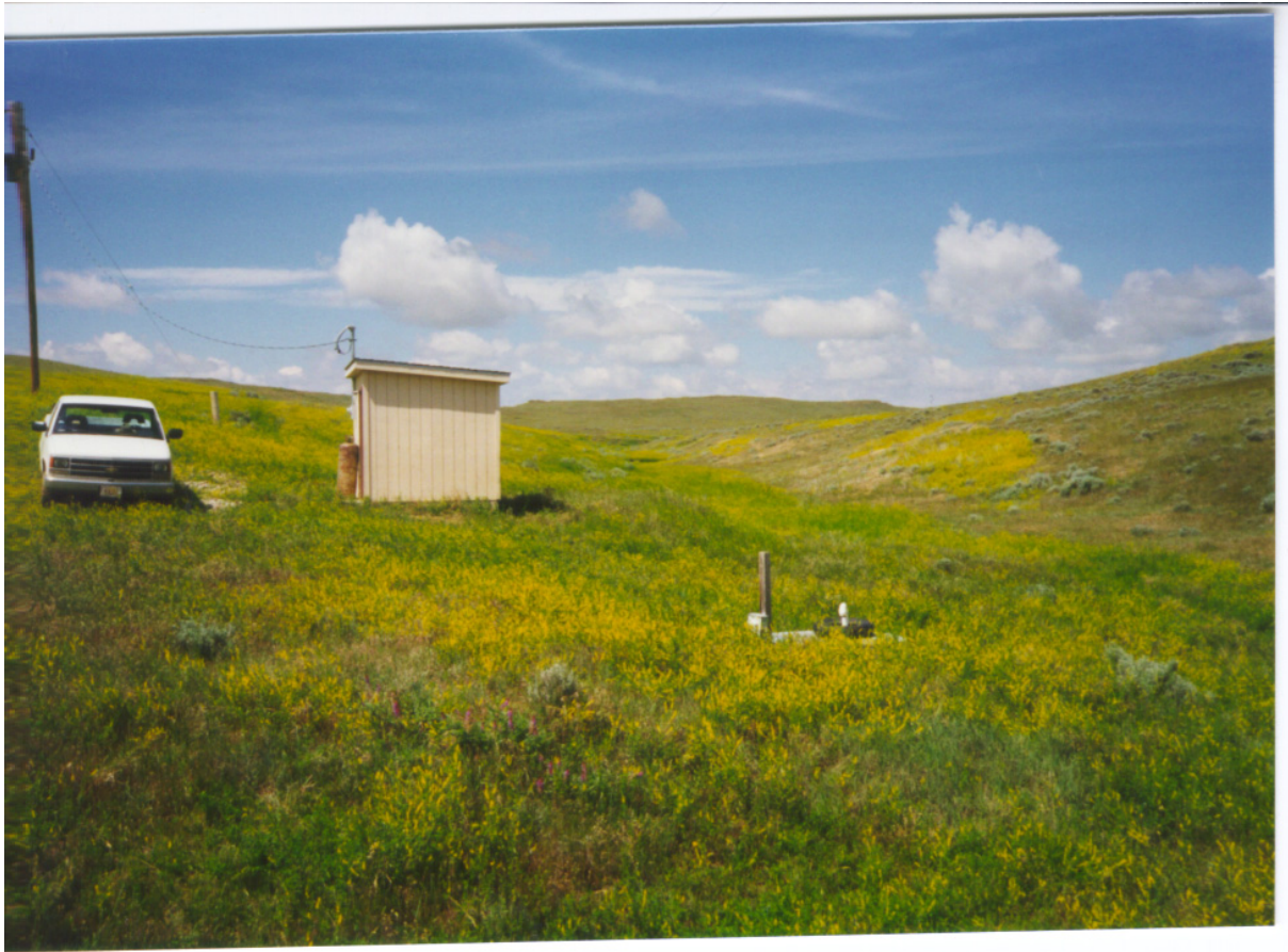
Photo 3. Looking west up coulee showing well in foreground and pump house. Colluvium covers the coulee bottom, the well is in the Fox Hills Sandstone, the hills in the background are Lance Formation bedrock. The infiltration gallery is buried behind the well and extends about 150 to 200 feet west, directly into the photo view.
