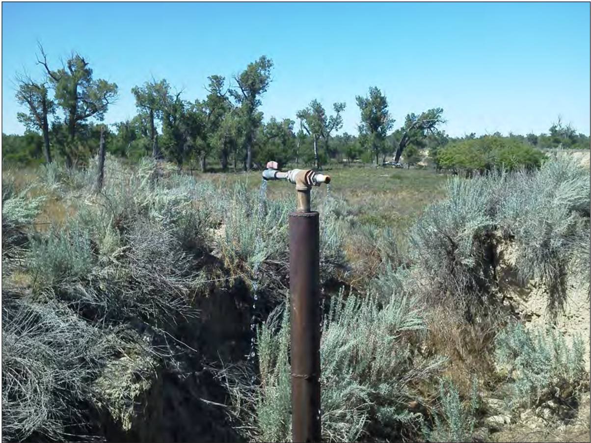
Figure 9. Erosion from continual flow has exposed more than 10 ft of casing.
