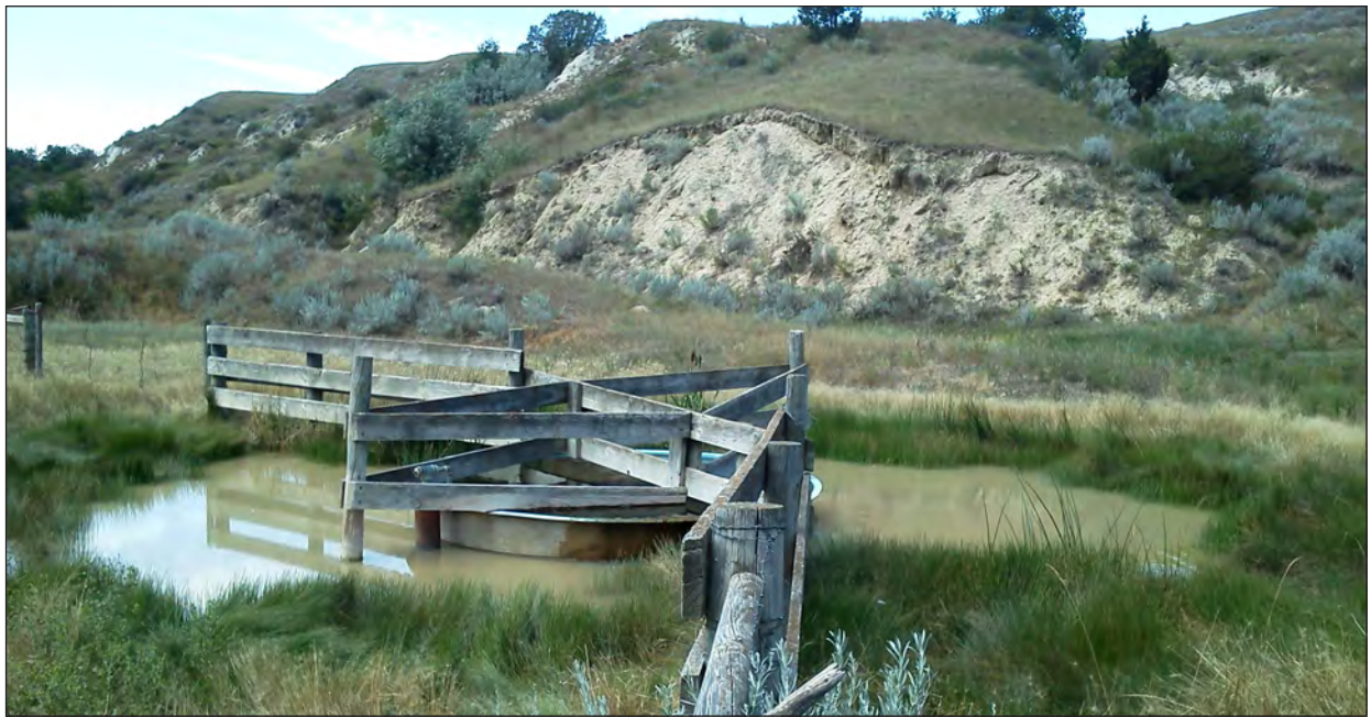
Figure 13. Leaky valves created a pond around the stock tank at well 35912.
