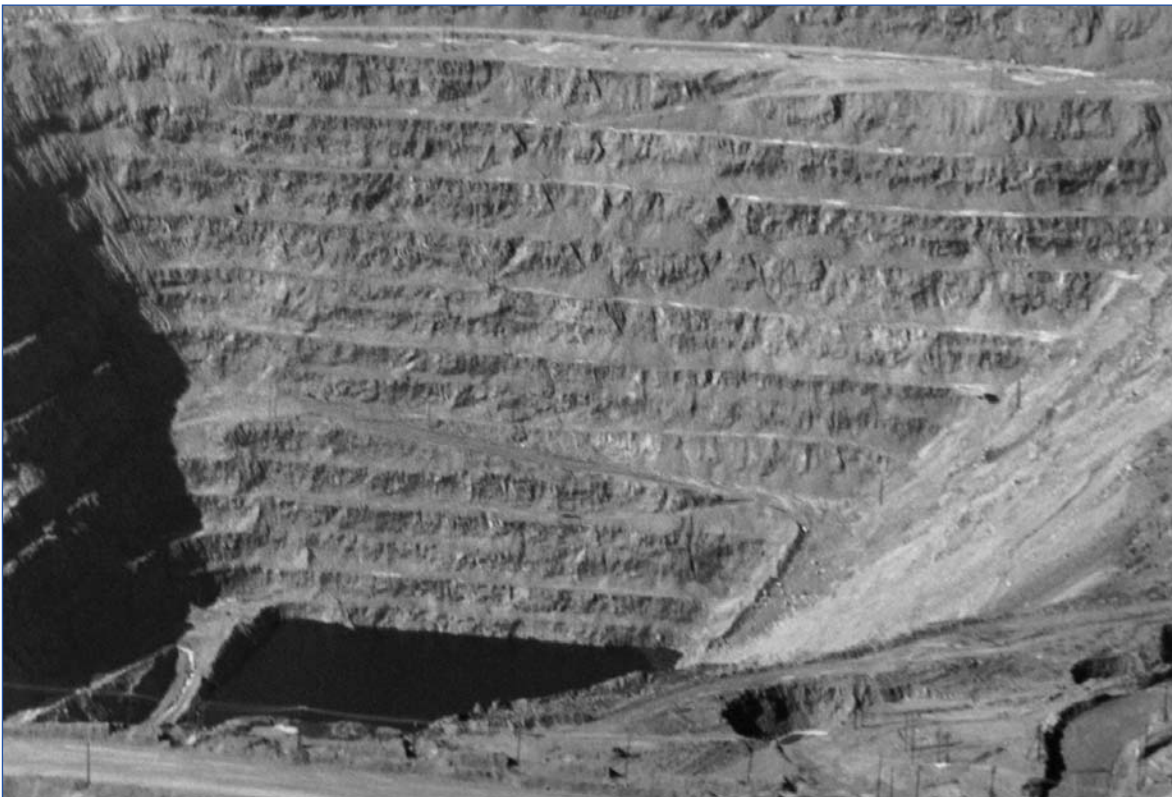
Figure 15. Standing water in the bottom of the Berkeley Pit, looking north, August 1983.
