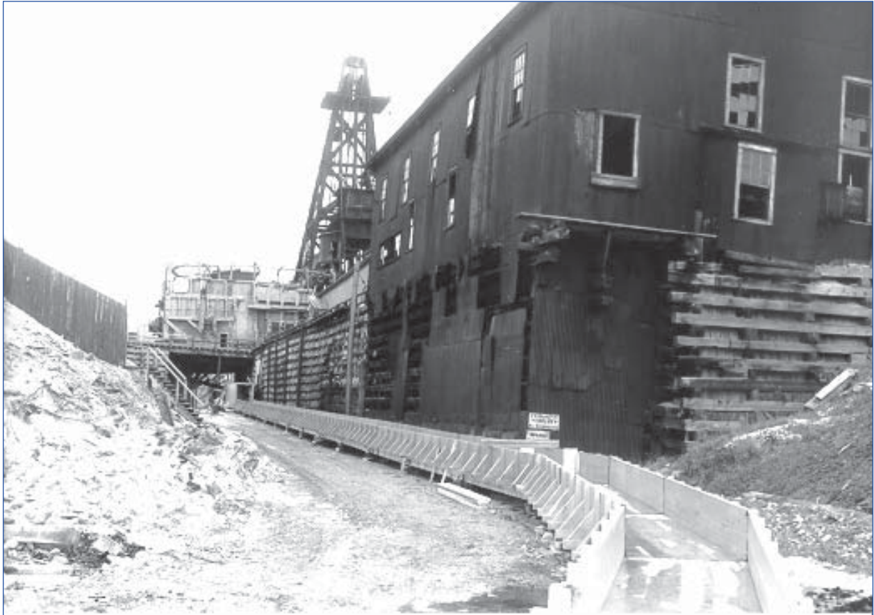
Figure 5. High Ore Mine and flume carrying underground mine water. (Photo courtesy World Museum of Mining, Butte, MT.)
