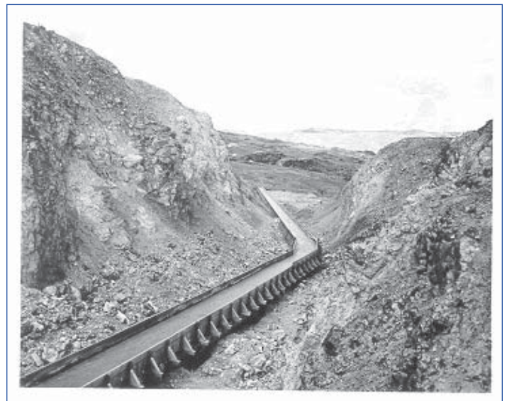
Figure 6. Flume carrying underground mine water from High Ore Mine to precipitation plant for recovery of copper. (Photo courtesy World Museum of Mining, Butte, MT.)
