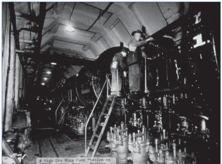
Figure 3. High Ore Mine pump station, 2800 ft level. (Photo courtesy World Museum of Mining, Butte, MT.)
