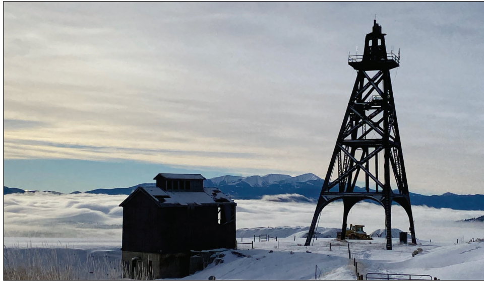
Headframe rising above the fog in Butte, Montana.
