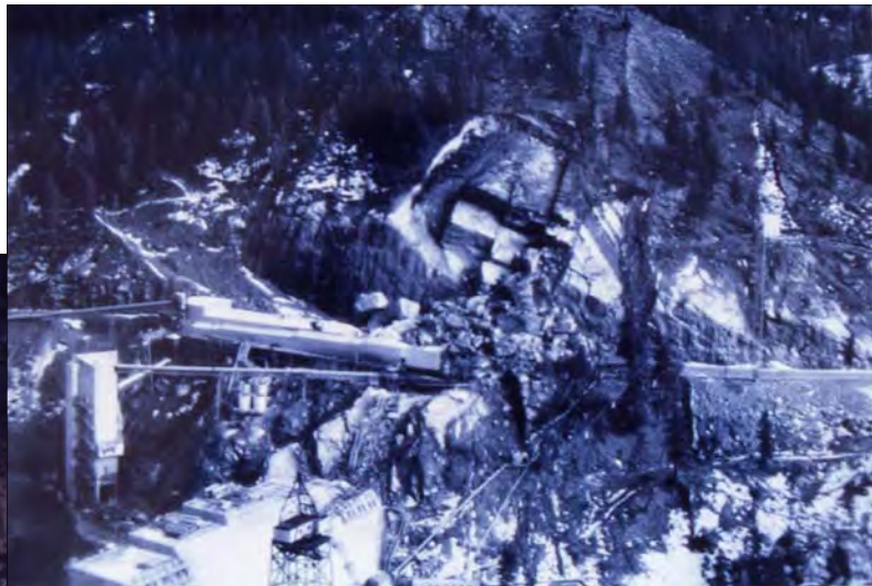
Fig. 2: The Libby Left Abutment slide on 31 January 1971. Photo taken on 2 February 1971. The contractor's cooling plant (ice house) is the horizontal building center, left. The concrete batching plant is the vertical building at lower left with the partly completed dam below. The slide occurred on a bedding plane fault and a near vertical E-W joint.
